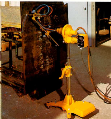
Horizontal position cutting with special leg assembly.
